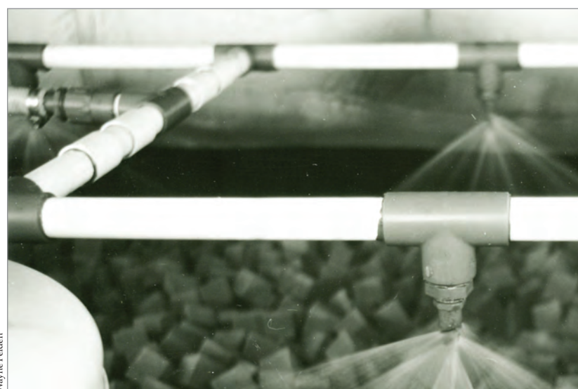
Figure 14. Trickling filter, artificial fixed film media; system in Gloucester, Massachusetts.
