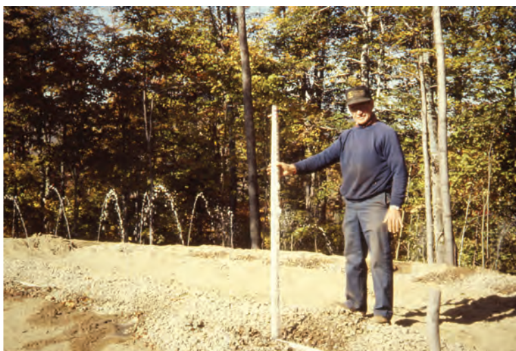
Figure 8. Pressure testing a low-pressure pressure distribution system (pressurized mound).
