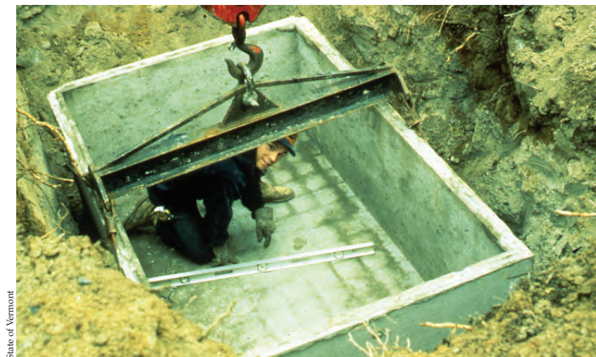
Figure 6. Bottom half of a concrete septic tank.
