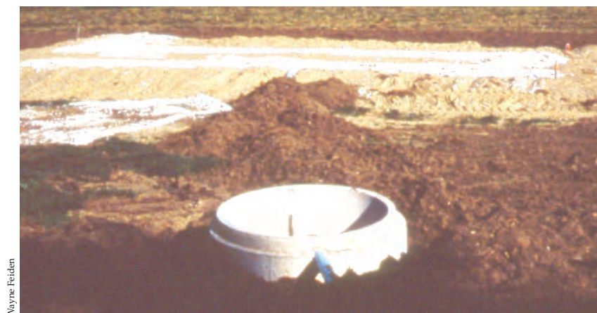
Figure 12. Siphon-fed pressurized mound system, Vermont.
