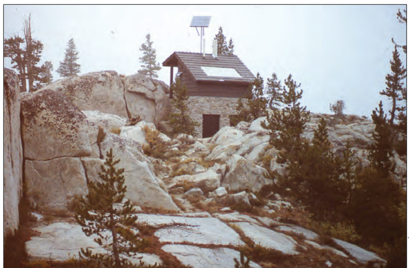
Figure 11. Alternative composting toilet in Sequoia/Kings Canyon, California.
