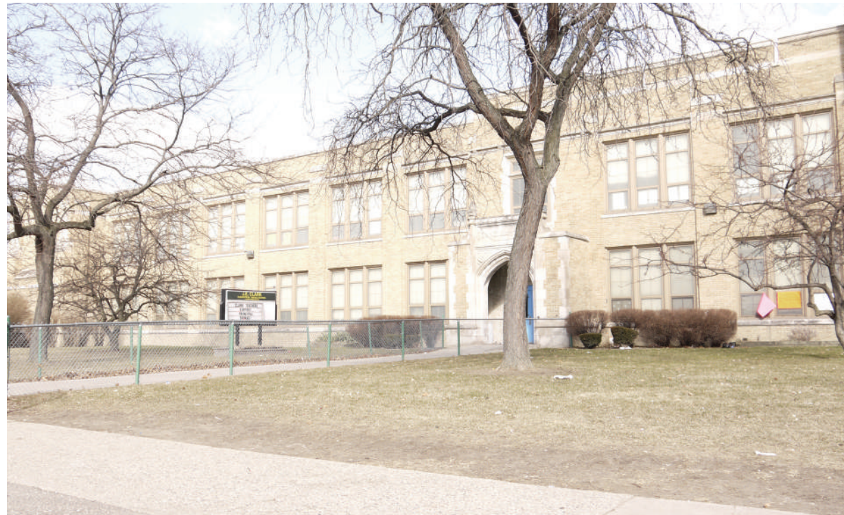
Figure 2.13: John Clark elementary school
