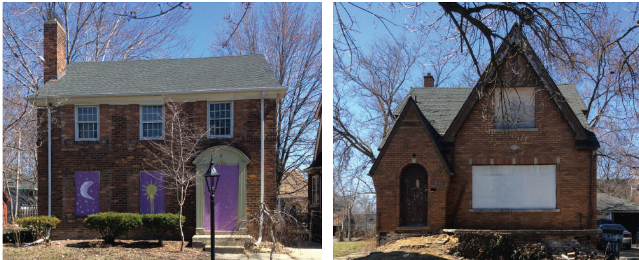
Figure 4.1: Potential homes to be renovated
