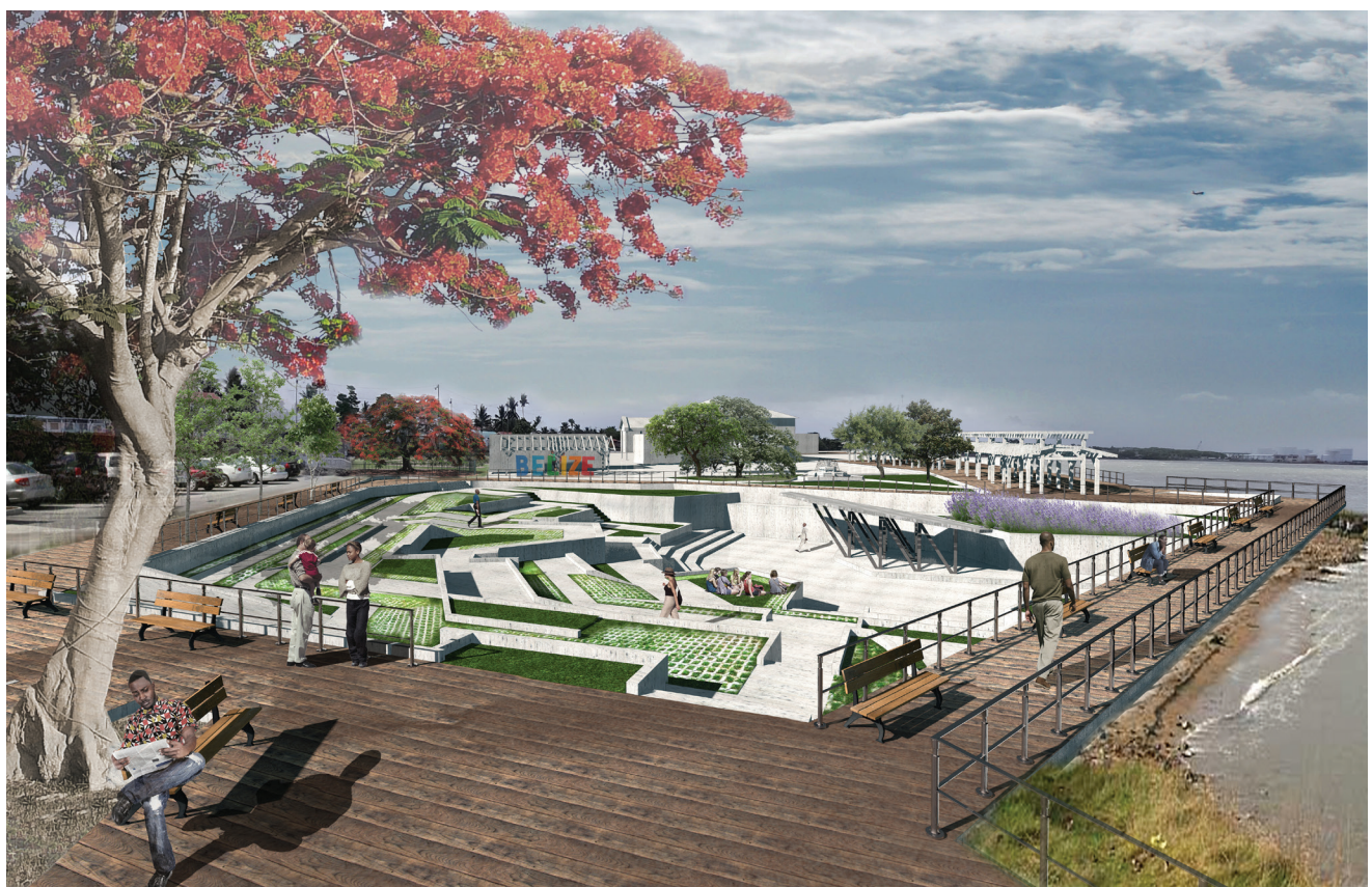
A representational rendering of the team's alternative site plan shows a reconfigured waterfront park that serves multiple functions and users. Cultural events and performances can occur in a new outdoor landscape amphitheater. During flood or storm events the lower sections of the amphitheater terraces can be flooded without significant damage. Source: Justin Moore, Francisco Jung, and CPAT Members
