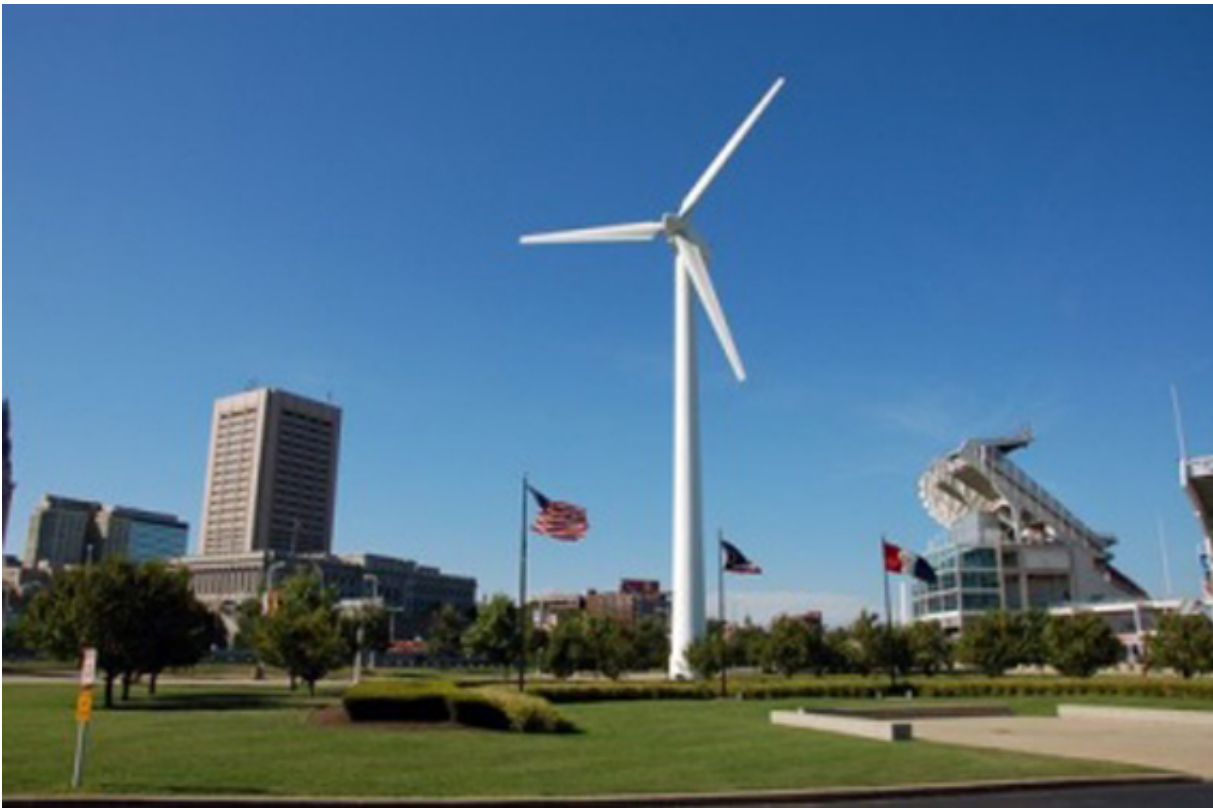
A wind turbine in downtown Cleveland. Photo courtesy DOE/NREL.
