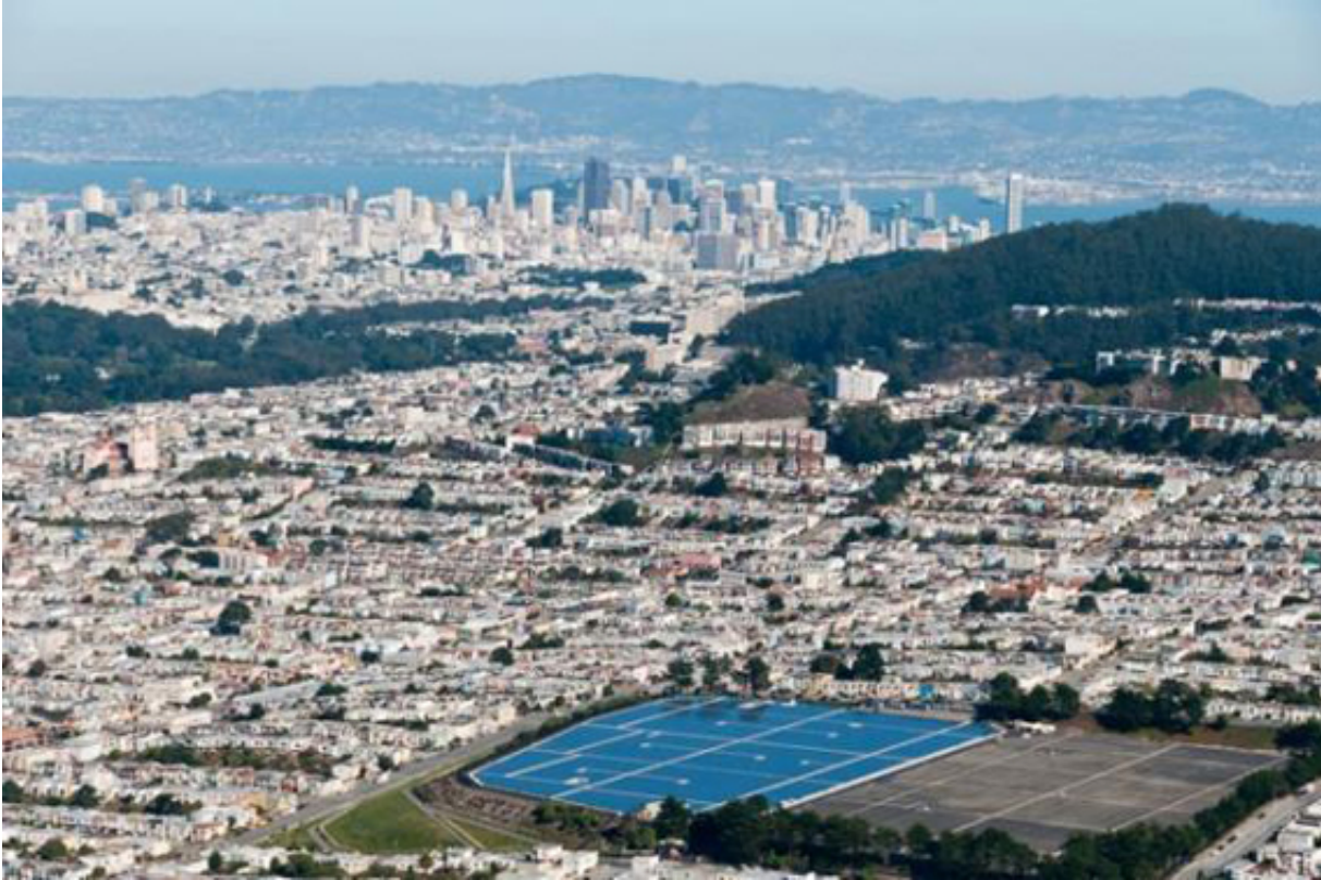
A 5-megawatt photovoltaic solar array sits atop the City of San Francisco's Sunset Reservoir. Photo courtesy San Francisco Public Utilities Commission.
