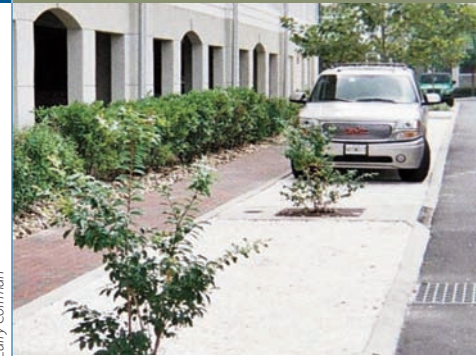
Tree box filters and infiltration parking areas along the roadway.
