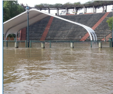
An outdoor amphitheater in Augusta, Georgia, designed to handle flooding from the Savannah River, floods after six weeks of constant rain in June and early July 2013. (Photo taken by Terri Turner, AICP.)
