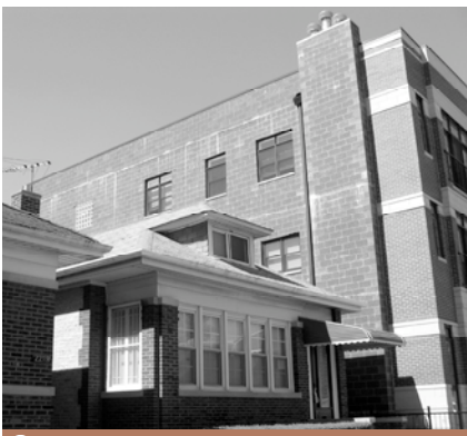
ⓘ Proper height and bulk regulations would have prevented the construction of this three-story condominium building in Chicago's Bungalow Belt.
