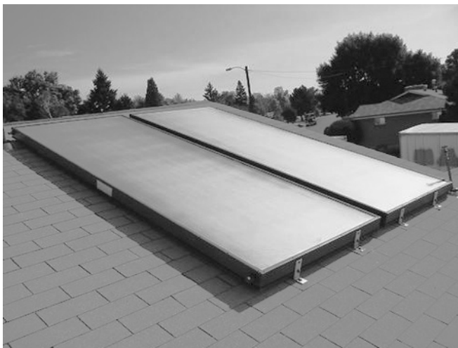
Solar hot water collectors on a Habitat for Humanity house in Denver.
