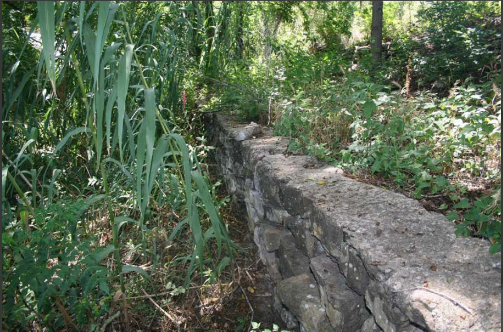
6- Stone retaining wall – south of W Court St
