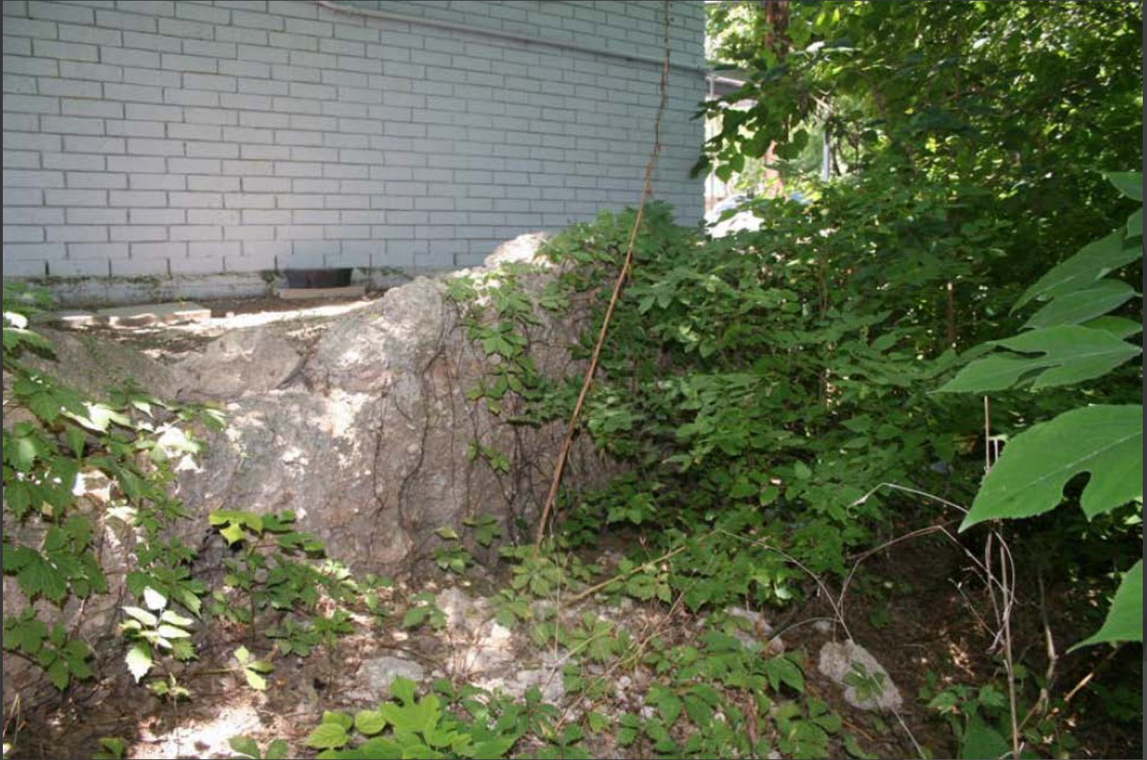
3- Limecrete retaining wall – west of N Guadalupe St
