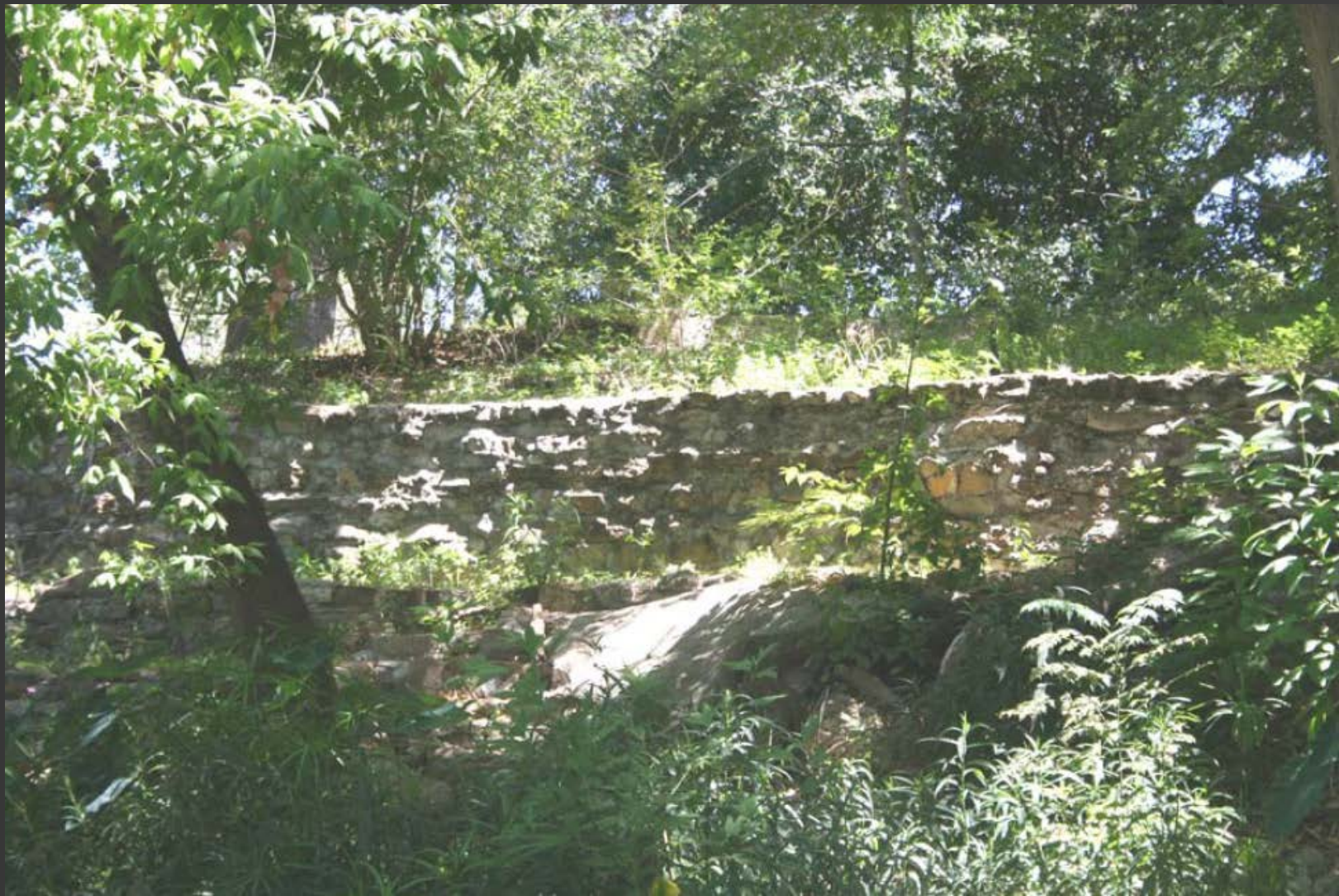
9- Stone retaining wall – north of W Nolte St
