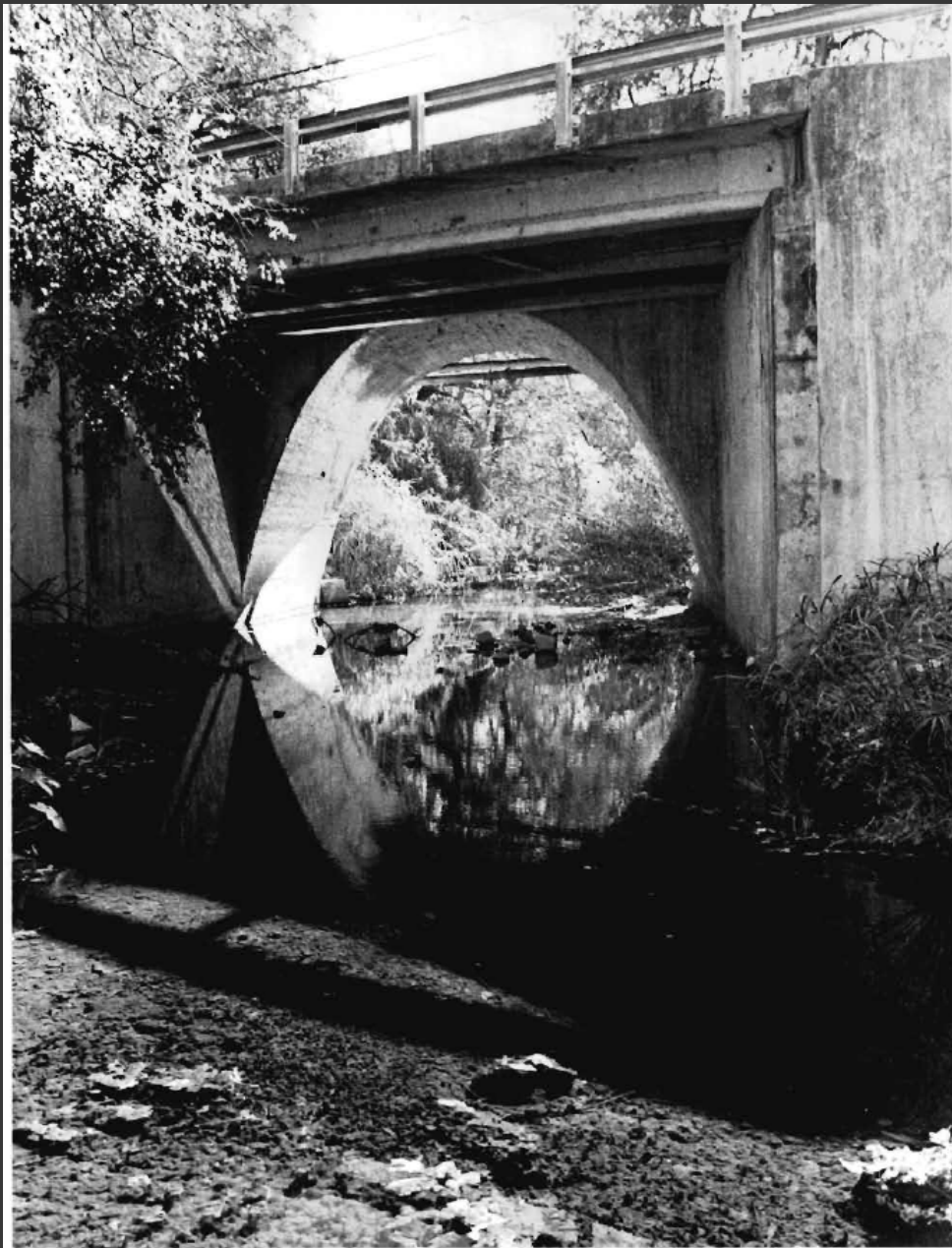
Nolte Street Bridge
