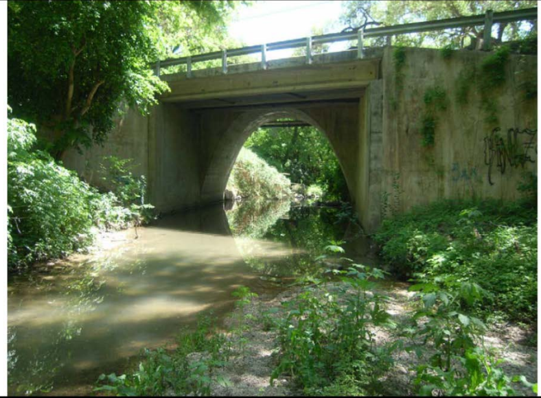
Photograph RIMG0095 April 11, 2007
