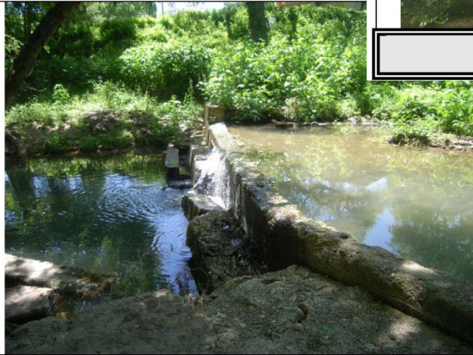
Photograph RIMG0099 April 11, 2007
