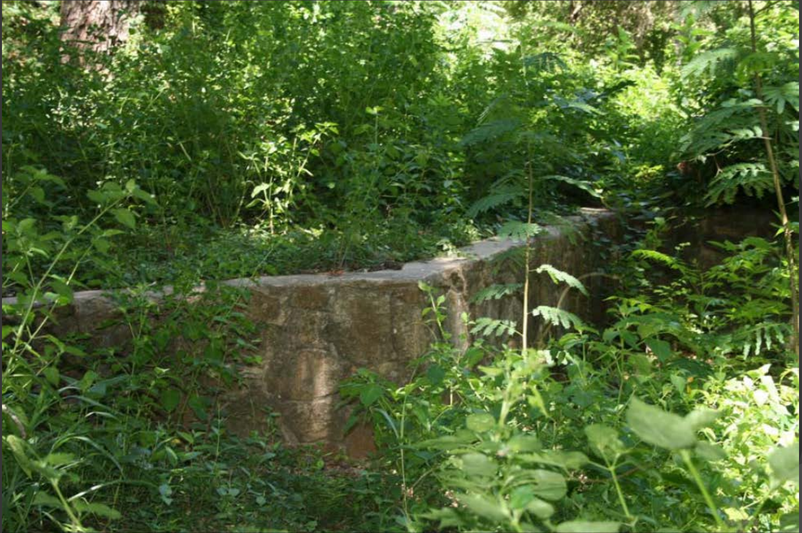
11- Stone retaining wall – north of W Nolte St
