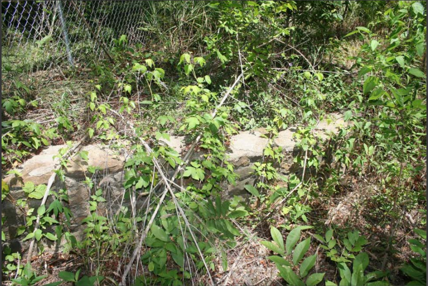
1- Stone retaining wall – west of N Guadalupe St
