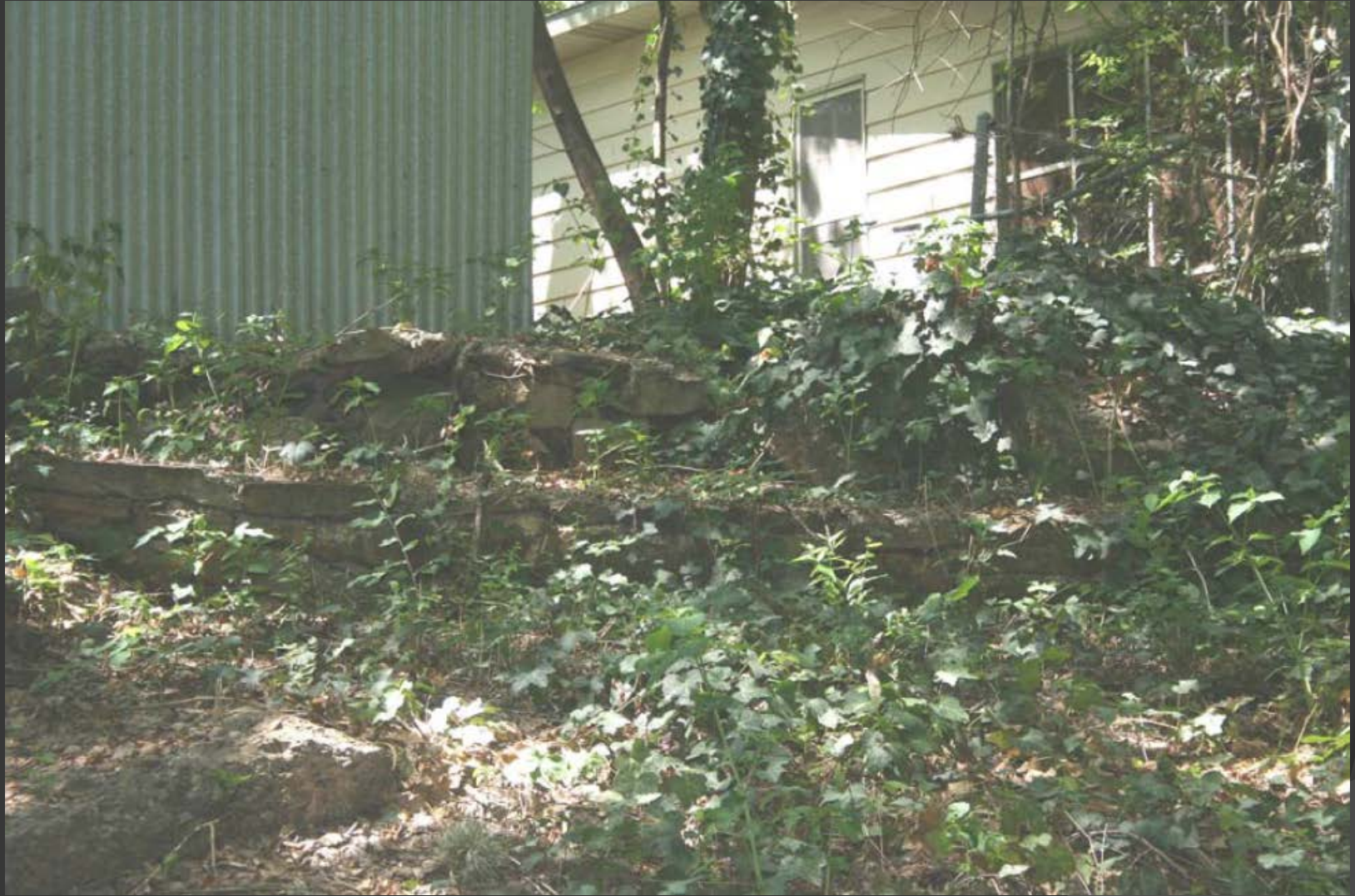
8- Stone retaining wall – north of W Nolte St
