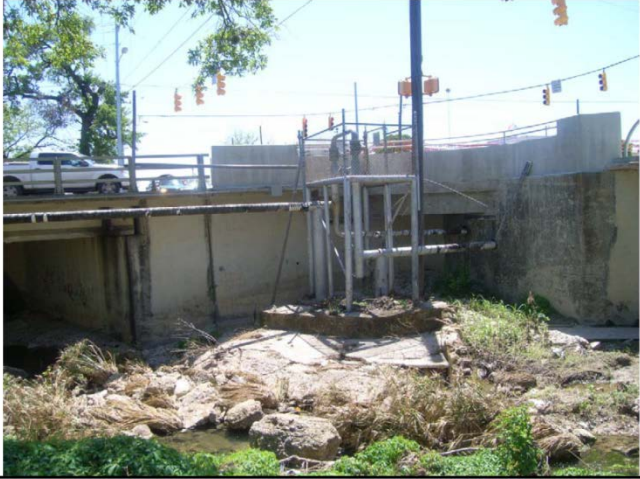
Photograph RIMG0090 April 11, 2007
