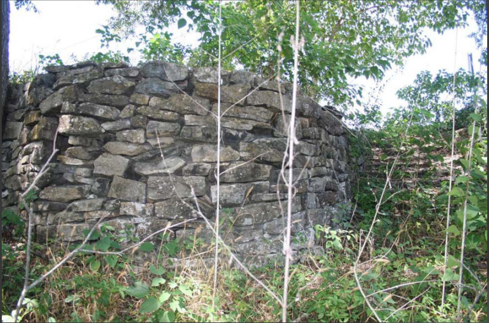
5- Stone retaining wall and steps— south of W Court St
