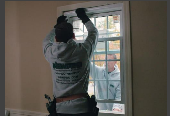
New windows & doors
