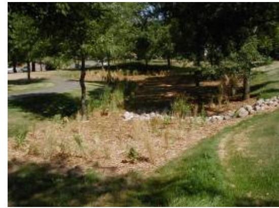
A rain garden in Dakota County, MN allows rain to return to groundwater in a cold, relatively dry climate.
