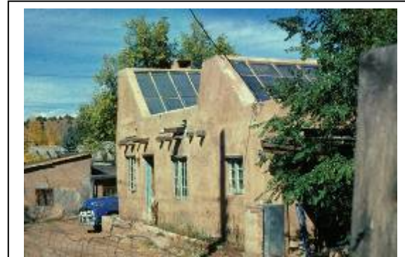
A sawtooth building in Arizona lets in north light and provides a south-facing surface for solar energy collection
