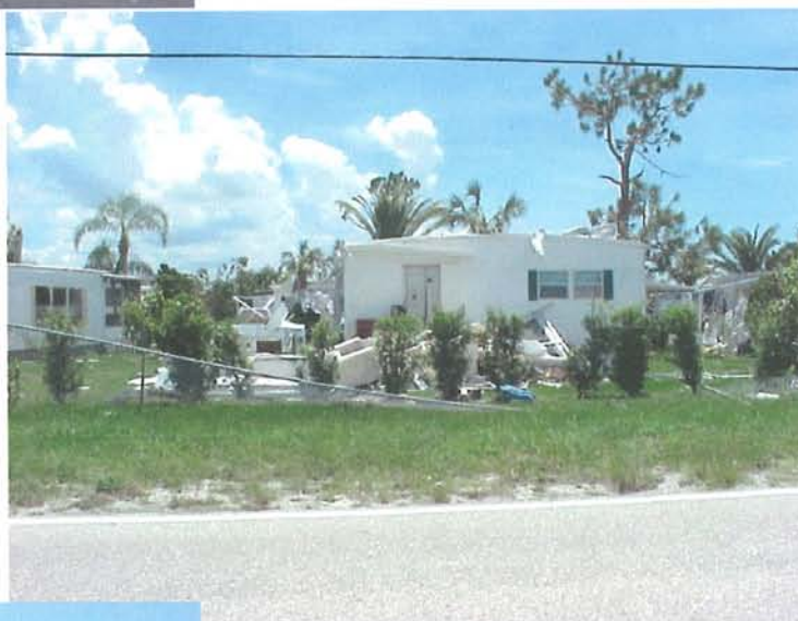
MOBILE HOMES SUSTAINED HEAVY DAMAGE IN PORT CHARLOTTE.
