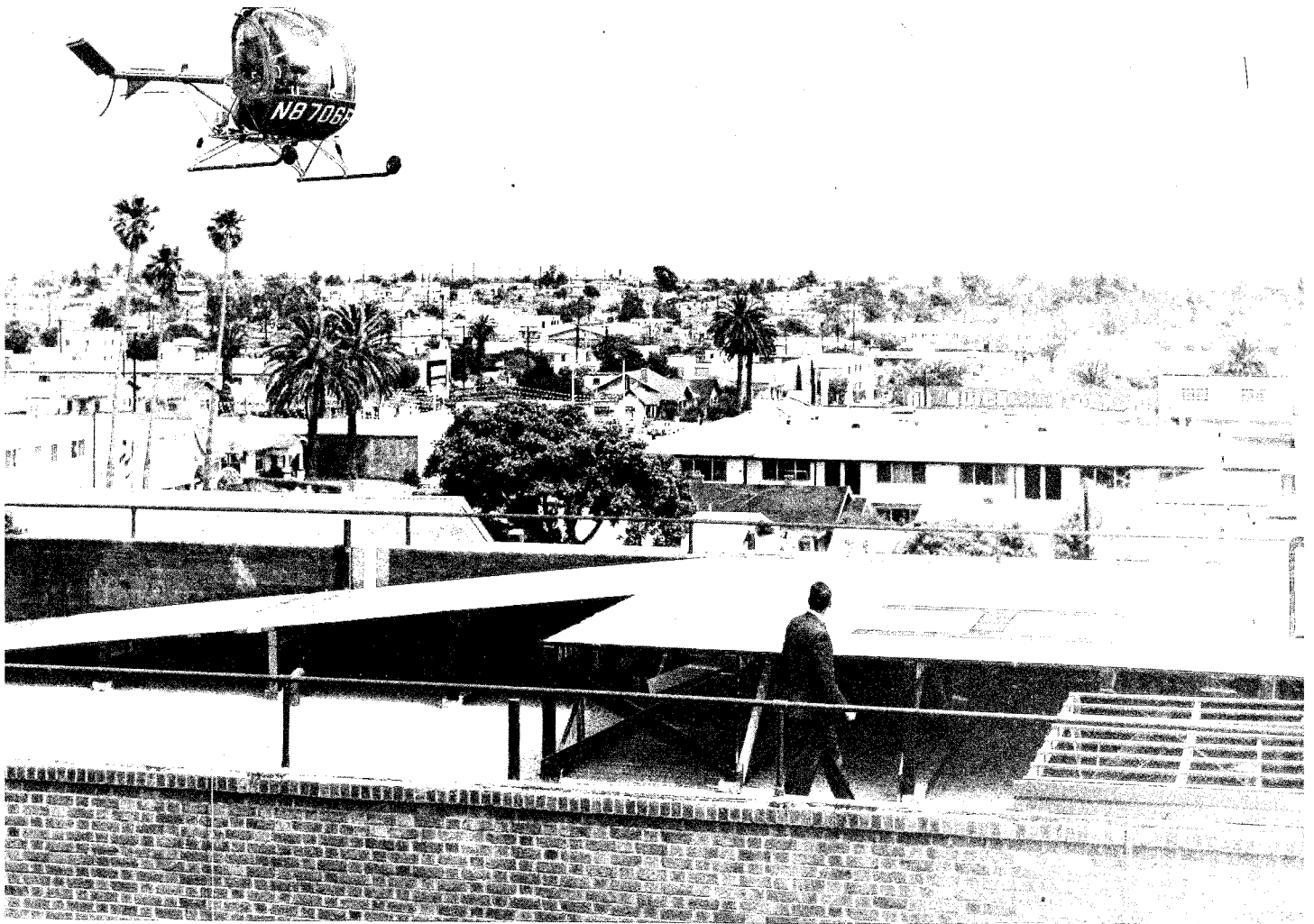
Rooftop landing area, Santa Monica Hospital, Santa Monica, California.
