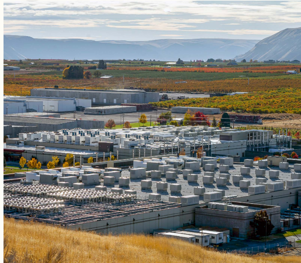
Data centers are responsible for approximately three percent of global electricity consumption and almost five percent of all the energy used in the U.S. Photo by Jovelle Tamayo/ The New York Times .
