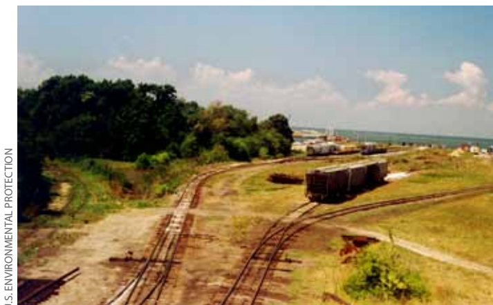
RAIL YARD AND DUMP SITE WAS CLEANED AND REDEVELOPED INTO A
