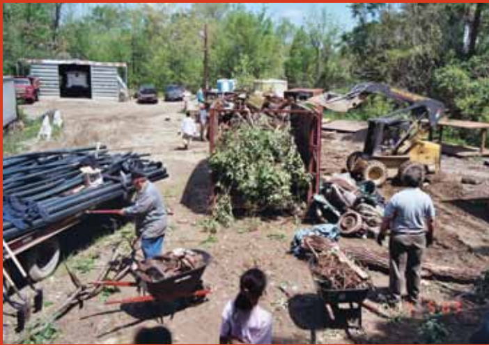
JUNK YARD CLEANUP ON SITE OF CLOSED CLEVELAND STATE HOSPITAL
