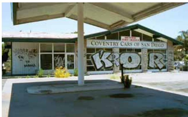
VANDALIZED GAS STATION IN SAN DIEGO, CALIFORNIA
