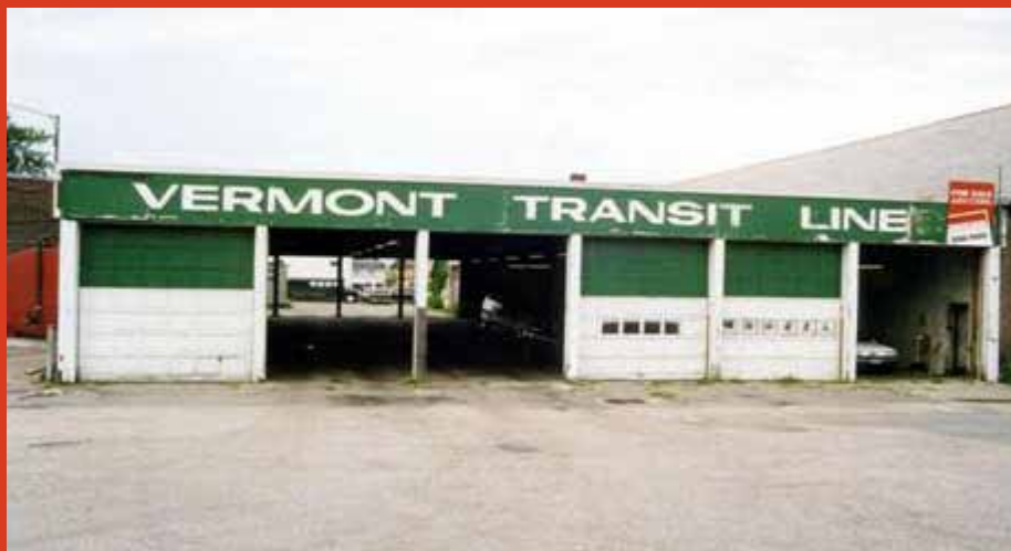
VERMONT TRANSIT BUS BARN BEFORE REDEVELOPMENT
