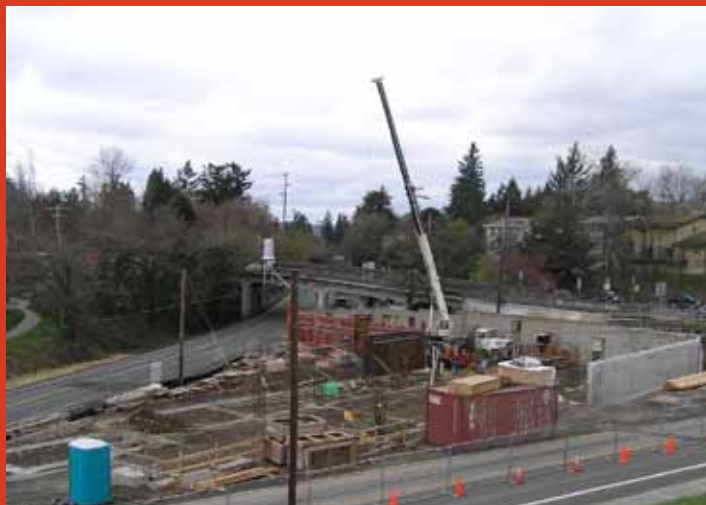
THE WATERSHED SITE UNDER CONSTRUCTION
