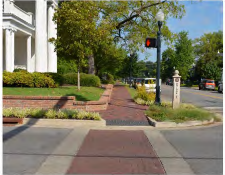
Bridge Street crossing
