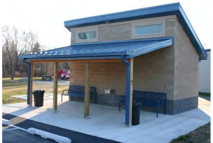
Example of open pavilion
