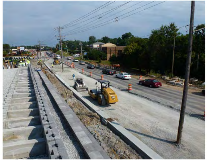
Hillsboro Street Improvement Project
