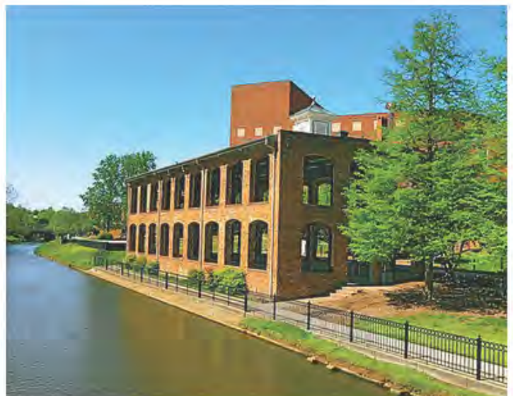
Example of floodable structure
