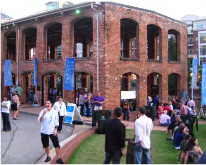
Example of floodable structure
