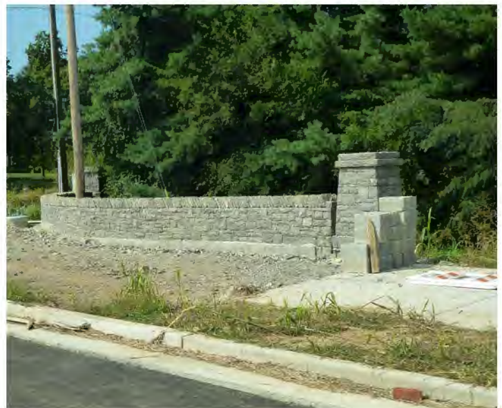
New 3rd Avenue culvert bridge
