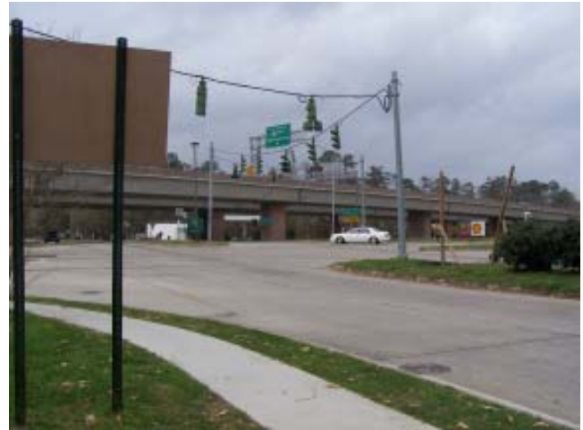
Major gateways such as Monroe and Causeway Approach should utilize wayfinding to help people locate notable destinations.
