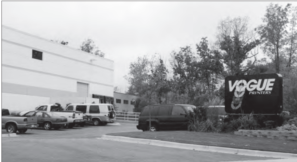
printing and publishing facility
