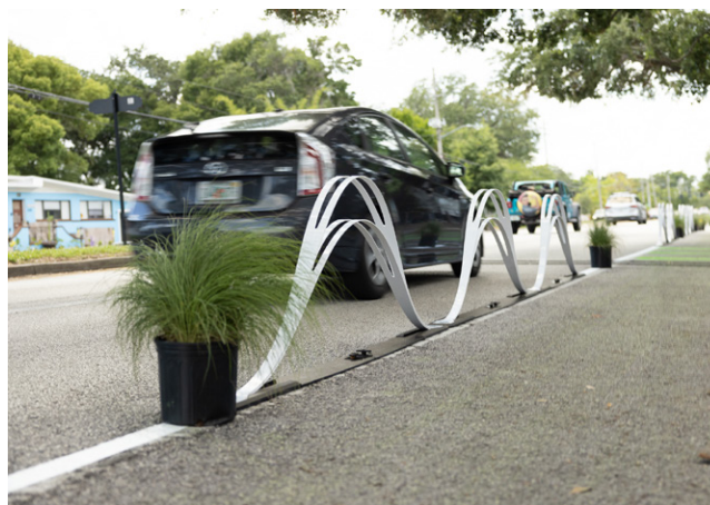
Figure 6.27. A protected bike lane with quick-build flexible separators and landscape elements (Kittelson)
