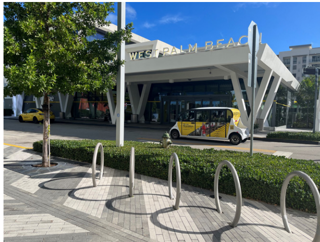
Figure 6.8. Angled on-street bike parking in West Palm Beach, with paver design helping to demarcate bike parking alignment (WGI, Inc.)
