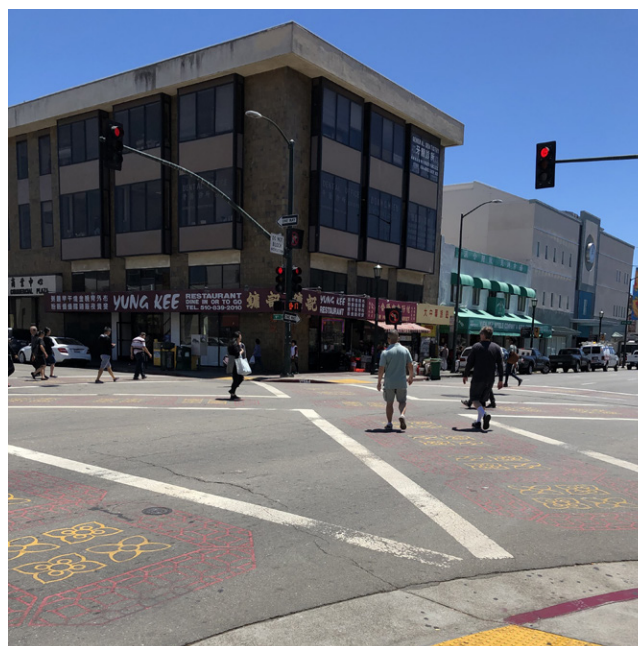
Figure 6.18. A scramble intersection, in which all traffic is stopped while pedestrians cross in all directions, including diagonally (Kamala Parks/pedbikeimages.org).
