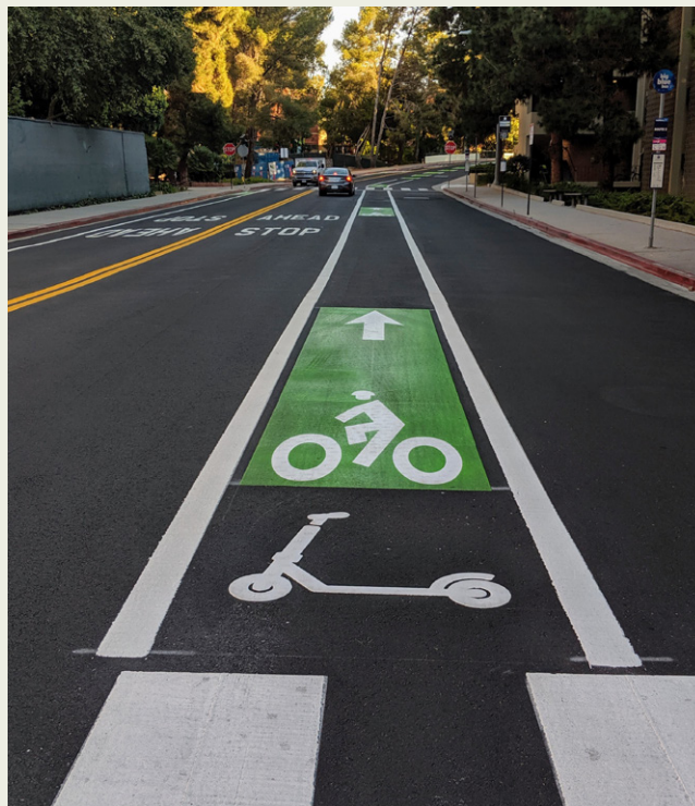
Figure 6.29. Micromobility lane using painted decals to designate space for both electric scooters and bicycles (Juan Matute)
