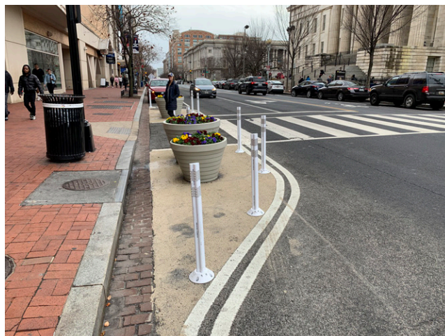
Figure 6.5. Portable planters add visual interest to quick-build installations (Andy Clarke, Toole Design)
