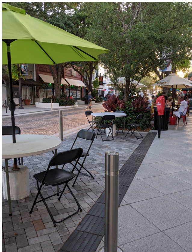
Figure 2.11. Clematis Street in West Palm Beach, Florida, combines a curbsless design and retractable bollards to facilitate programming (WGL, Inc.)
