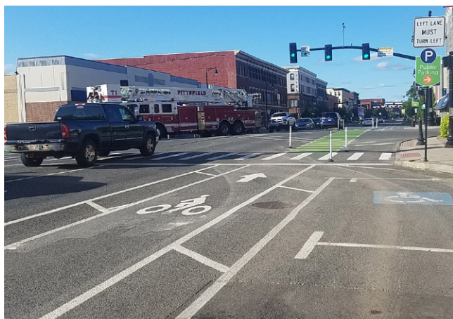
Figure 6.26. A bike lane with painted buffers from the travel lane and on-street parking (Kittelson)
