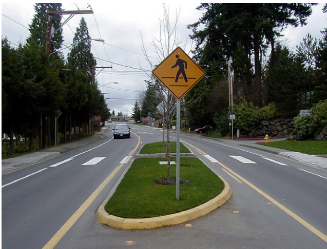
Figure 6.14. Example of a raised median island with a midblock crosswalk (Dan Burden/www.pedbikemages.org)
