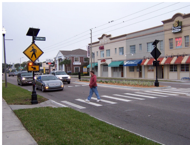
Figure 6.16. Rectangular rapid flashing beacon (RRFB) at a crosswalk (Michael Frederick/ www.pedbikeimages.org )
