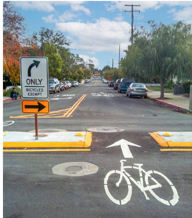
Figure 6.15. A diverter directs cars to a right-hand-only turn but allows bicycles and pedestrians to continue straight (Adam Fukushima/pedbikemages.org)
