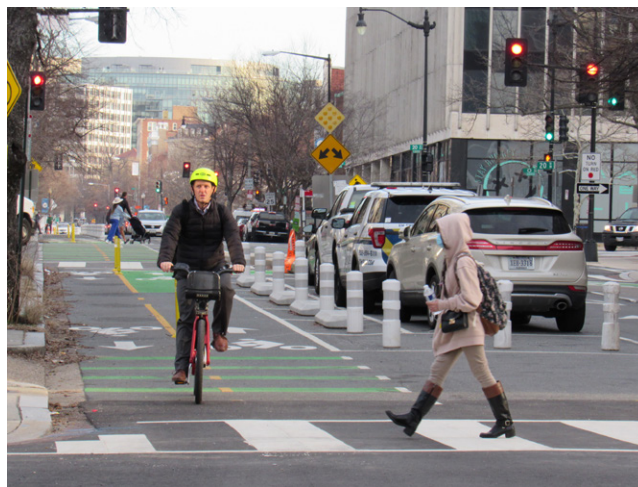
Figure 6.28. Protected bike lane between the sidewalk and on-street parking on 15th Street in Washington, D.C. (Andy Clarke/Toole Design)
