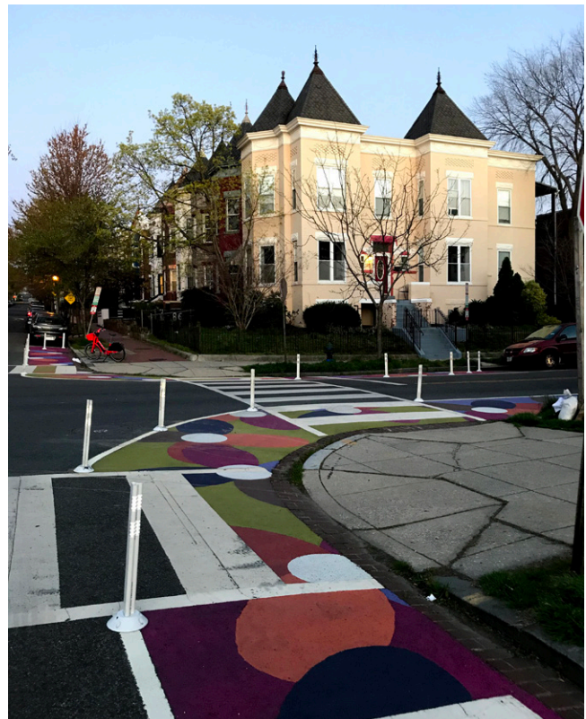
Figure 10.4. A quick-build installation in Washington, D.C., that uses art and flexposts to reduce the speed of turning cars (Kittelson)
