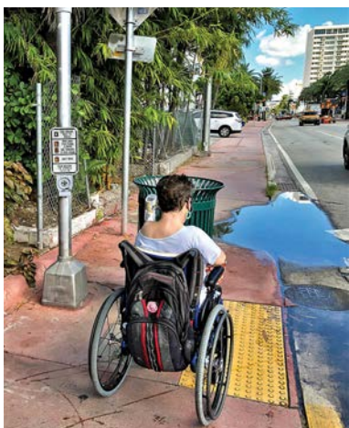
Curb ramp issues include too-narrow ramps, garbage cans and street furniture on the sidewalk, and poor drainage.
