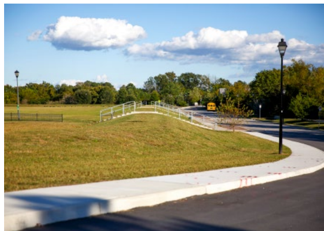
Clockwise from above: The tidal gate along Kimball Terrace; a project map; and the berm that helps to protect the Chesterfield Heights and Grandy Village neighborhoods as part of the Ohio Creek Watershed Project.
