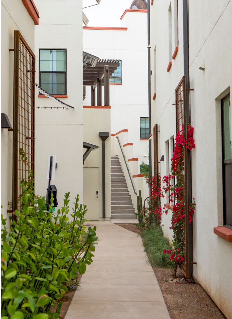
Above and right: Culdesac draws on elements of Mediterranean design. The placement of buildings, walkways, and shared spaces creates a quiet coziness.
