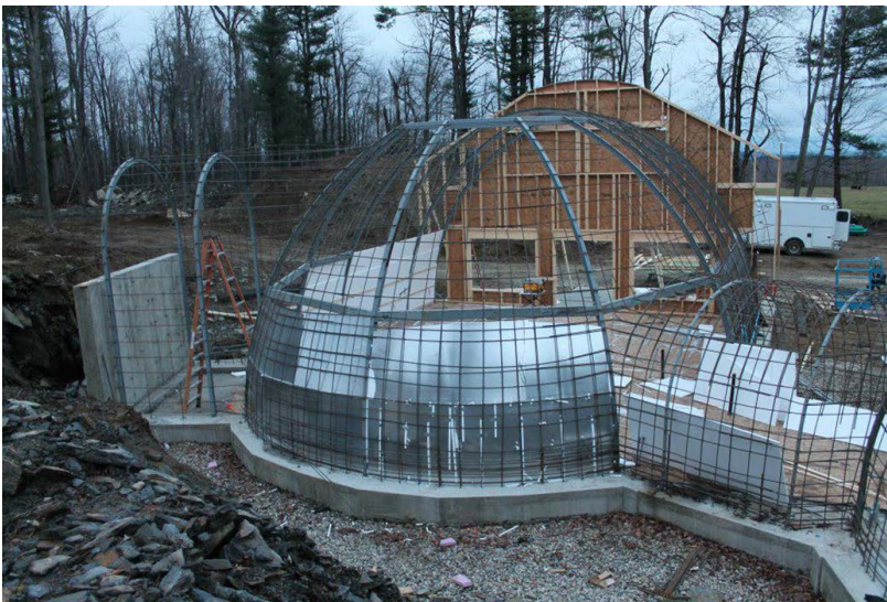
An earth-shelter home under construction in Hawley, Massachusetts (Credit: Formworks Building)
