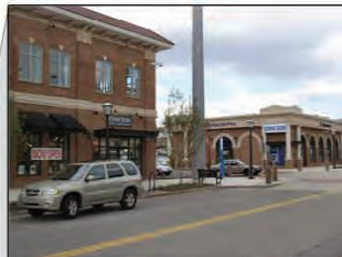
Street treatment on large retail sites is an important factor in creating a different type of retailing that is very different from the large surface parking lots like those at the Front / Gause intersection. Curbside parking provides a neighborhood feel with storefronts on the sidewalk providing lots of interaction and making people feel safer at any time of day.
