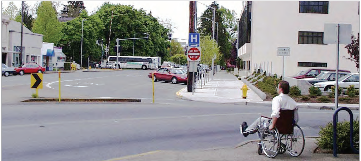
Figure 7.21. Free-flowing turn lanes can create pedestrian hazards.
