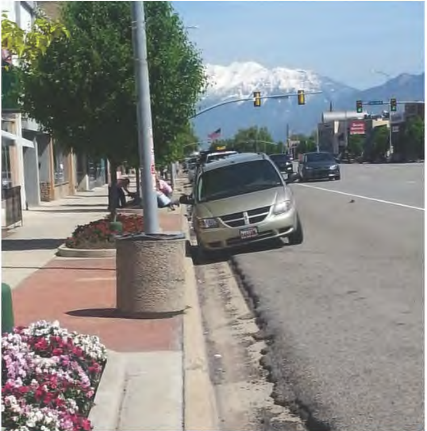
Asphalt buildup on Main Street
